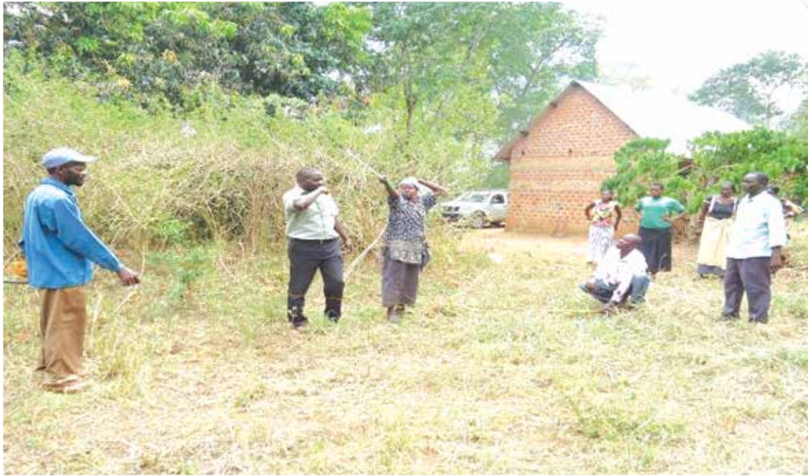
Figure 7 Members of the Kyabutaika Innovations platform, Kakooge Sub County, Nakasongola district guides Mr Simon Ogwal (AfrII) on the site they have selected and cleared to locate the housing structure for the FMT. Mrs Mary Mutyaba, the leader of the group, shows Simon the direction the sun sets and rises so as to guide the layout of the housing structure
