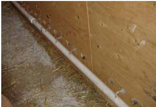
Photo 3.3 PVC pipe and holes are drilled through the plywood to the feeding area.
